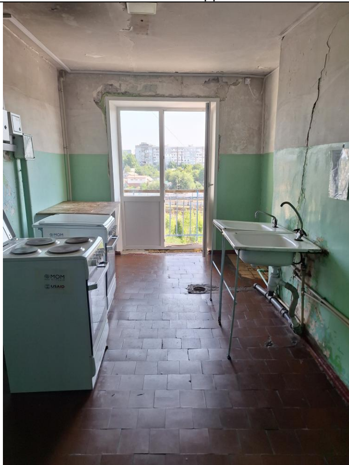
9th Floor BEFORE / ДО
